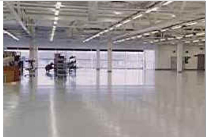
Sealed and Heat Welded PolyStat becomes an impervious seamless static control floor.
