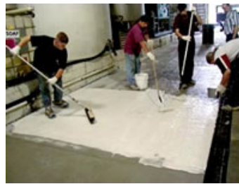
8. Carefully scrub SG1 or SG2 into the pores with a long handled scrub brush.
