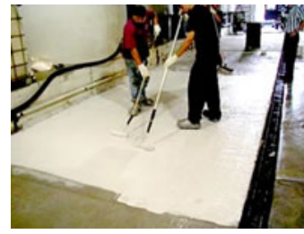
9. Follow with a roller to achieve a uniform coverage, and broadcast sand as necessary. Consult product data sheet.
